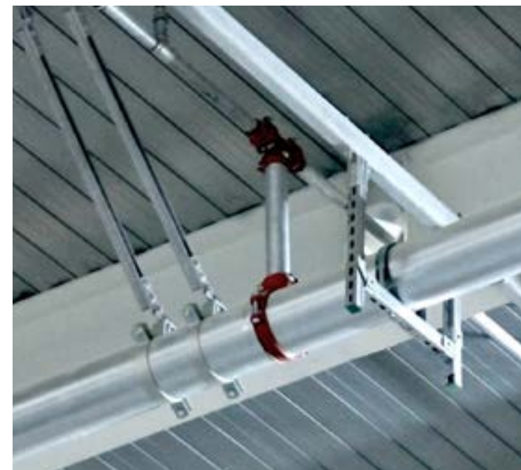
Seismic bracing
